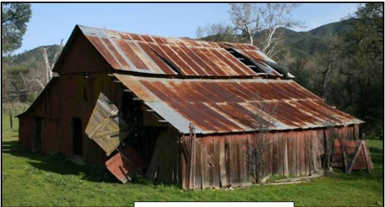
Merle Ranch Barn, Northwest Corner
