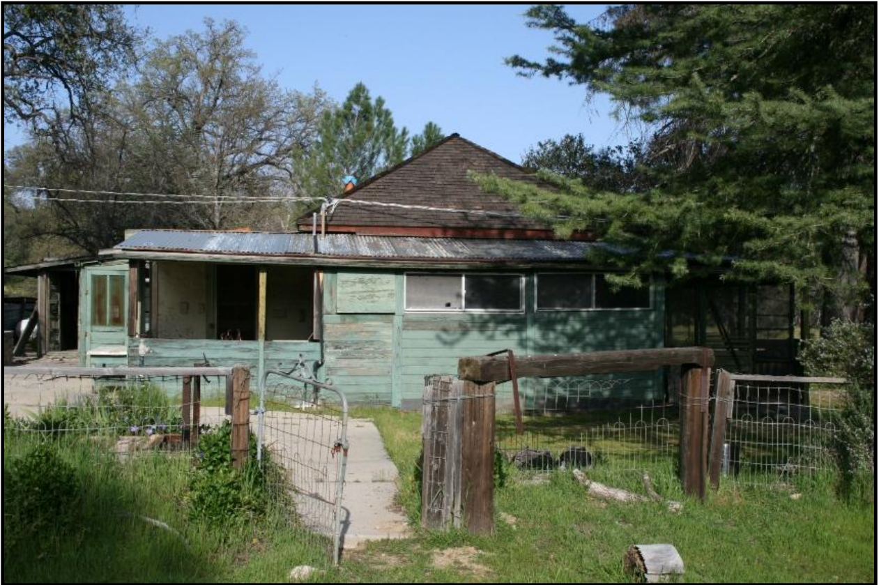
Merle Ranch Headquarters, West Elevation
