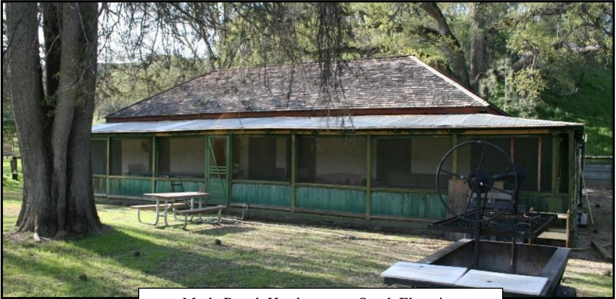
Merle Ranch Headquarters, South Elevation
